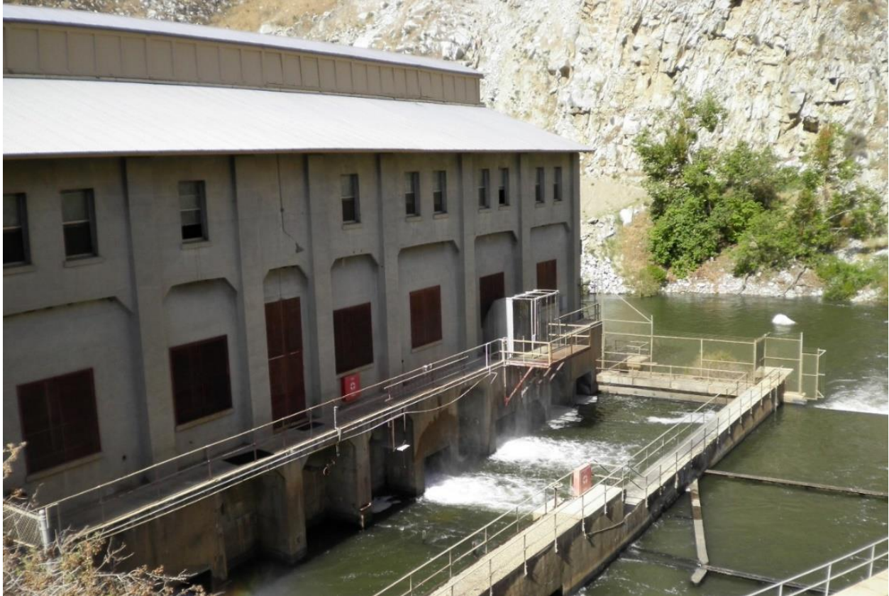
Photo A-8. Kern River No. 1 Powerhouse and Tailrace.
