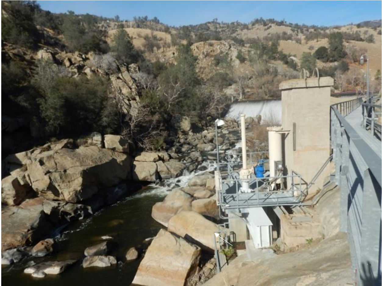
Photo A-5. Slide gate valve house at the downstream end of the sandbox (approximately 700 feet downstream of the Diversion Dam at the head of the flowline).
