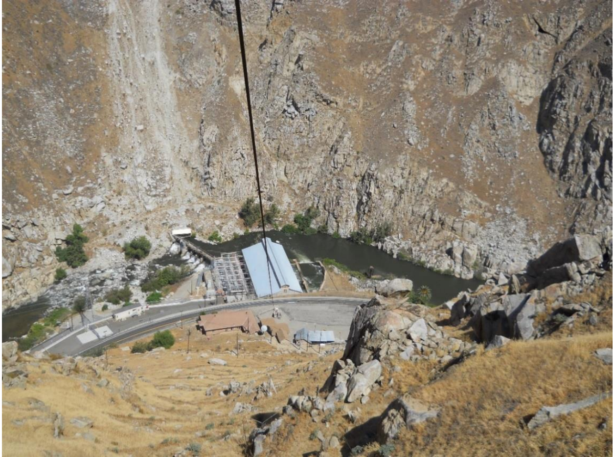
Photo A-11. View of the Kern River No. 1 Powerhouse and Switchyard and Forebay Operations Area as seen from the Skip Hoist Upper Landing. The skip hoist cable is visible in the foreground.
