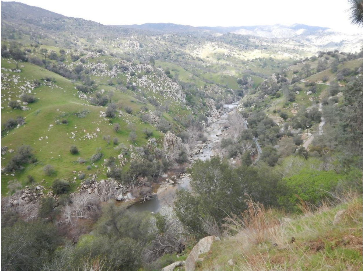
Photo A-1. Democrat Dam and elevated steel walkway on top of Flume No. 1 as seen from SR-178.
