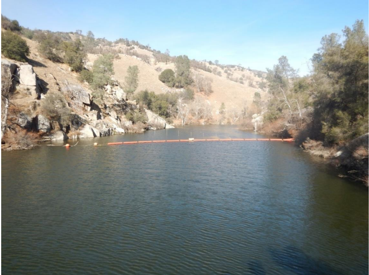
Photo A-7. Democrat Dam Impoundment and buoy line, looking upstream from the dam.
