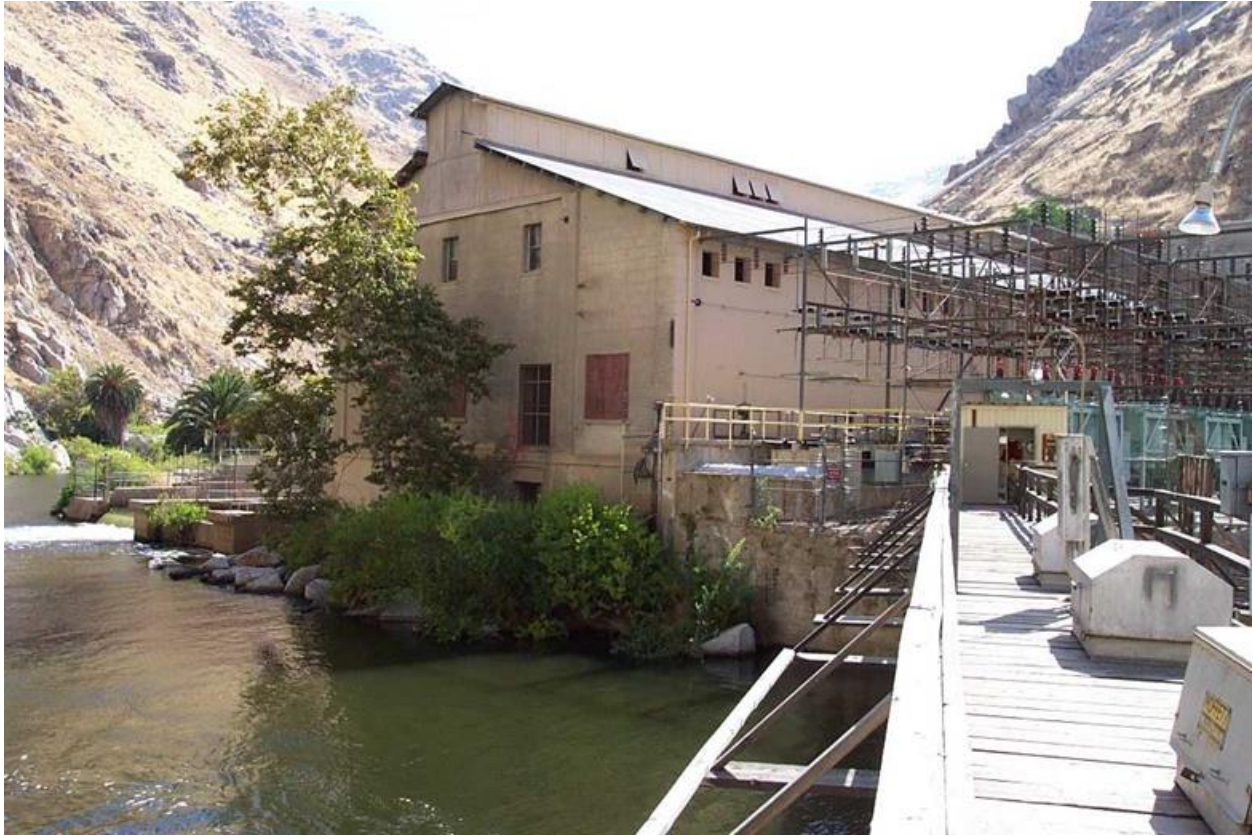
Photo A-9. Kern River No. 1 Powerhouse and Switchyard.
