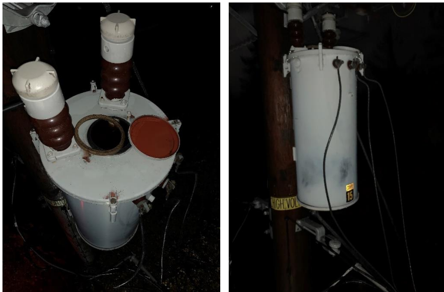
Figure 57: Failed Transformer was the first Permanent Ground Fault at Arrowhead
