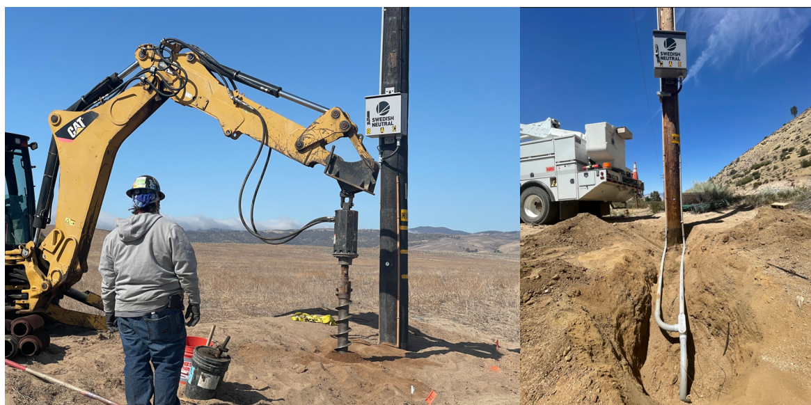
Figure 26: Deep Grounding Electrode Installation
